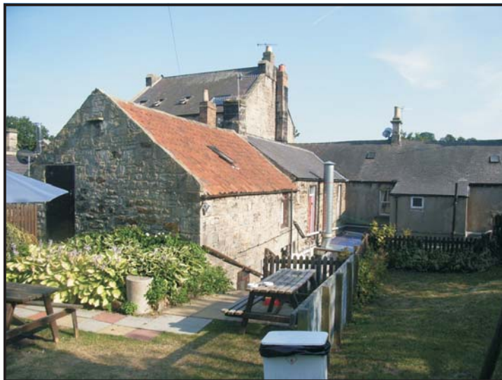
Illus. 40: The rear of the Turks Head, with possible former brewhouse to left of view.
